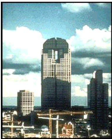
Texas Commerce Bank Tower, Dallas, USA
