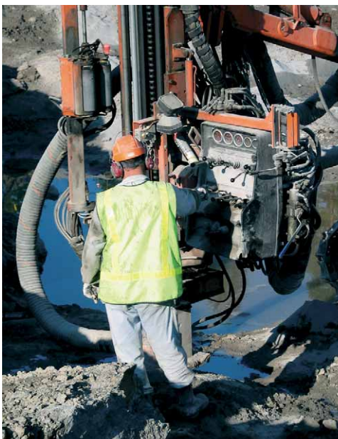
Excavation in June 2004
