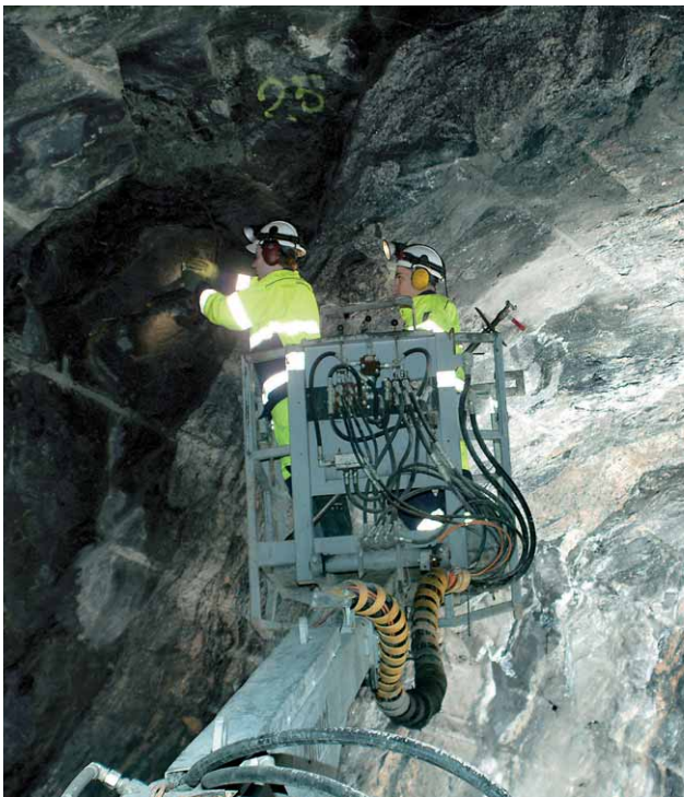
Mapping of the tunnel rock surface
