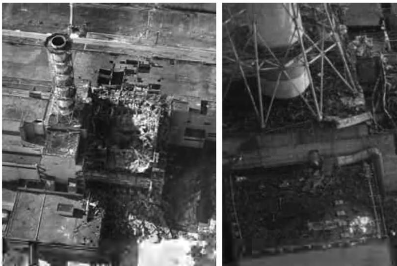
*A segment of fire fighters' work area # 2 - the roof nearby Unit 4. Fragments of the reactor core are visible - the ones thrown by the explosion onto the roof of unit B where the ventilation stack is installed. The photo was taken from the North; the destroyed reactor room of Unit 4 may be seen in the right part of the left photo, on the left, the roof of the reactor room of Unit 3 is visible. The right photo provides a close-up view of one of the roofs.*
