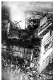
*The view of the northern side of the destroyed reactor unit building. Releases of water vapour and radioactive products are visible.*
