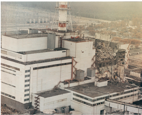
Fig. II.1: The damaged reactor
