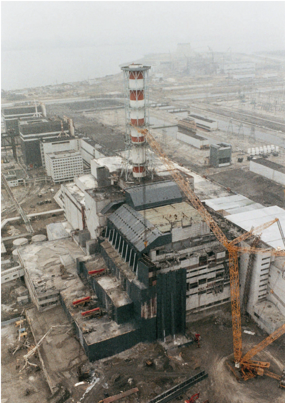
Fig. II.2: Construction of the sarcophagus
